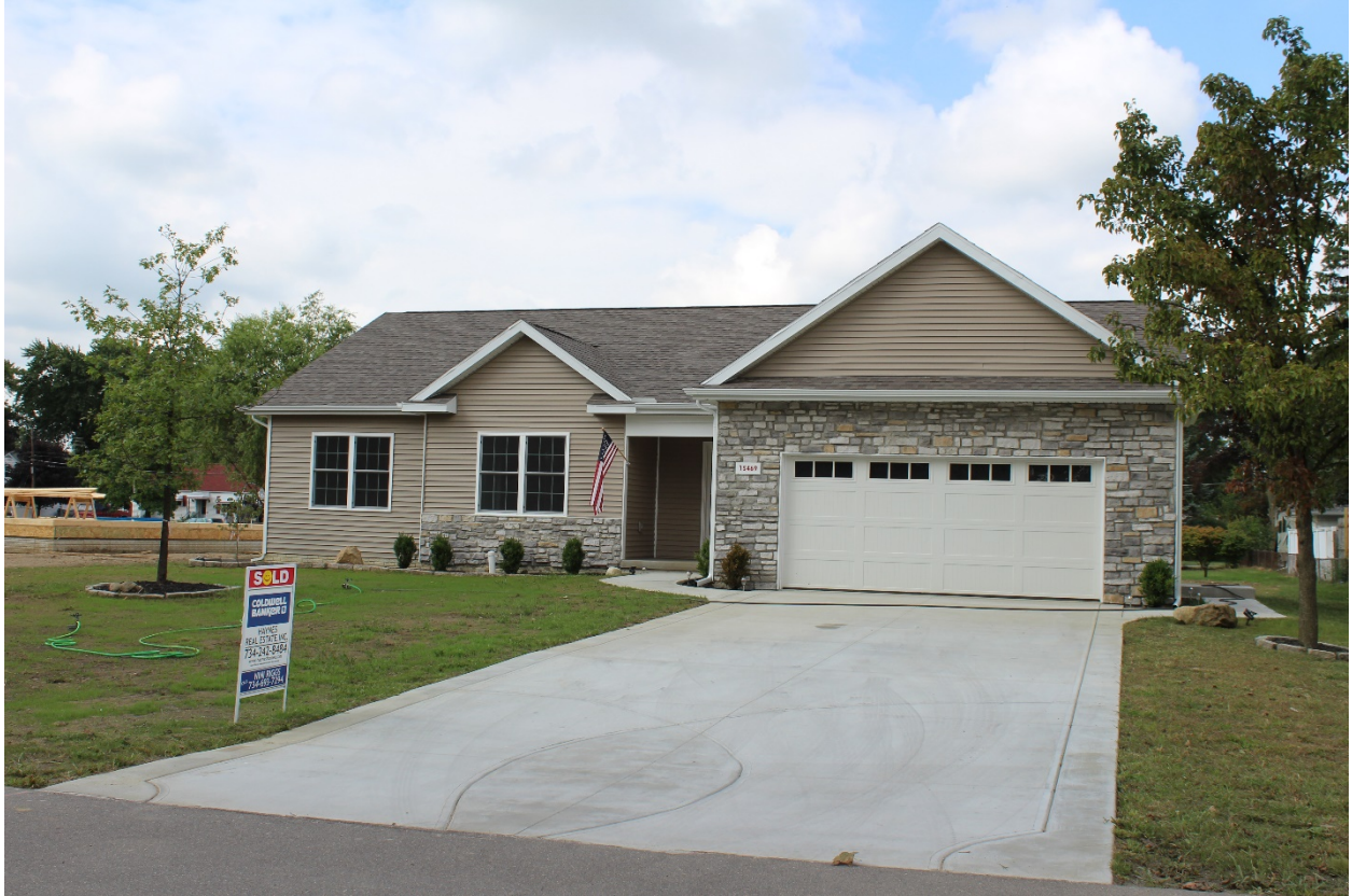
Closing on Trojan Build #1, 15469 Charles Street, was held on September 16, 2019.
